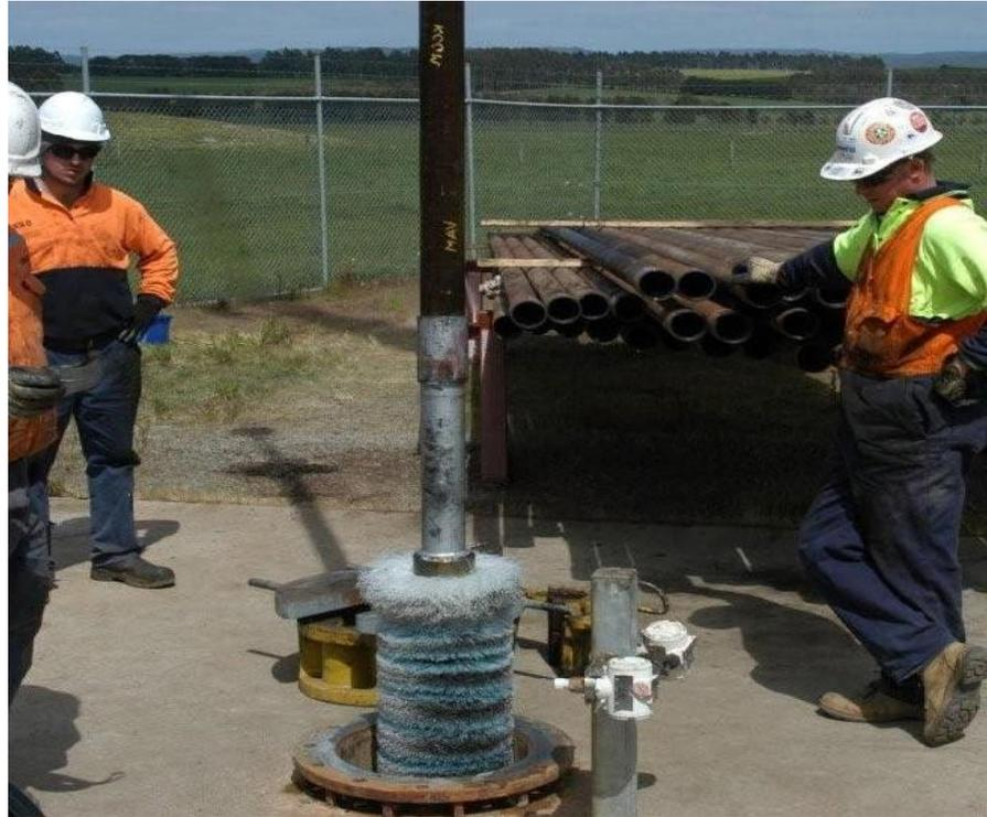
Rig washing is a necessary part of the drilling operation, not just for safety of the rig floor workers but also for the containment and sustaining the environment around the drill site. In the case of some recent gas plays like the Barnett Shale, drilling rigs are operating in neighborhoods, near schools, city buildings and airports.
